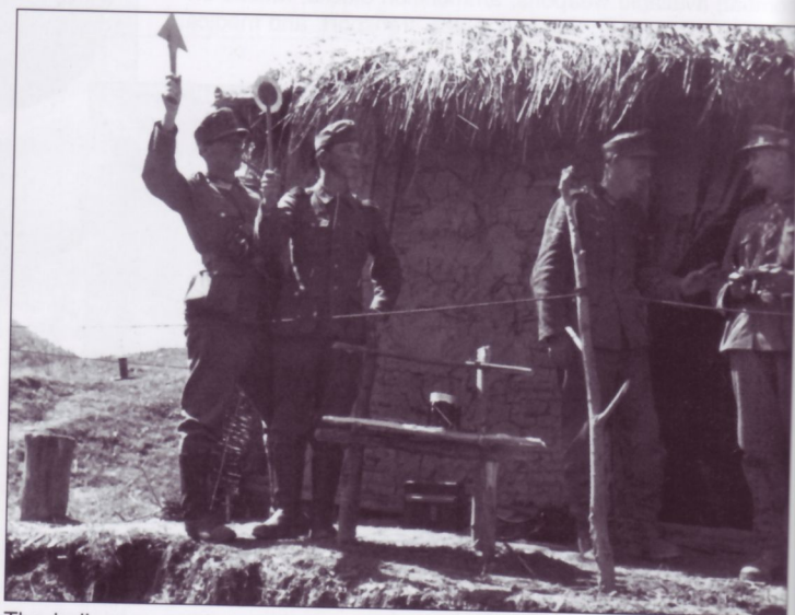
The balloon ground control station supervised the charging of the balloon with hydrogen, determining the amount of ballast sandbags necessary for the desired altitude and expected temperatures, transmitted ascent and descent orders, and monitored wind speed and direction. Orders were transmitted using signs.
