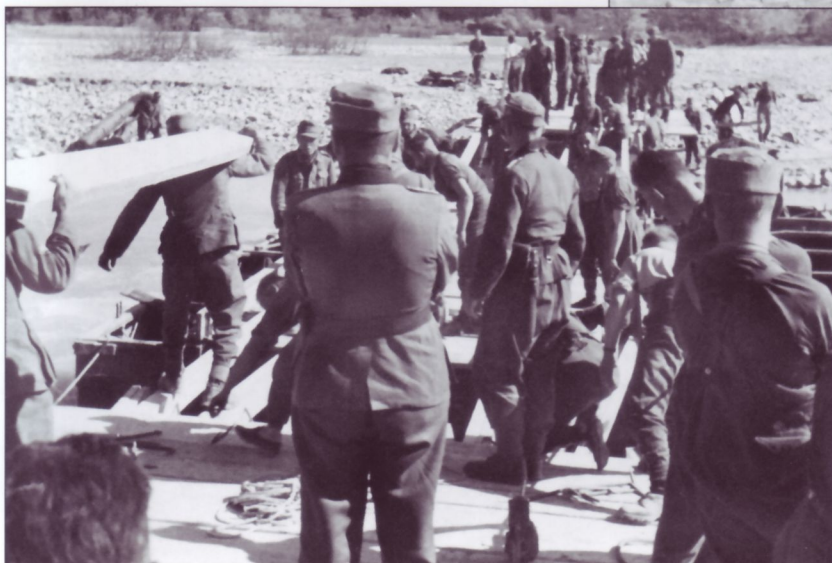
A Gebirgsjäger general officer looks on as pioneers complete a wooden trestle bridge with the end bridging a deeper channel supported by four pontoons. The light wooden pontoons are for the bridge equipment "C" (Brückengerät "C").
